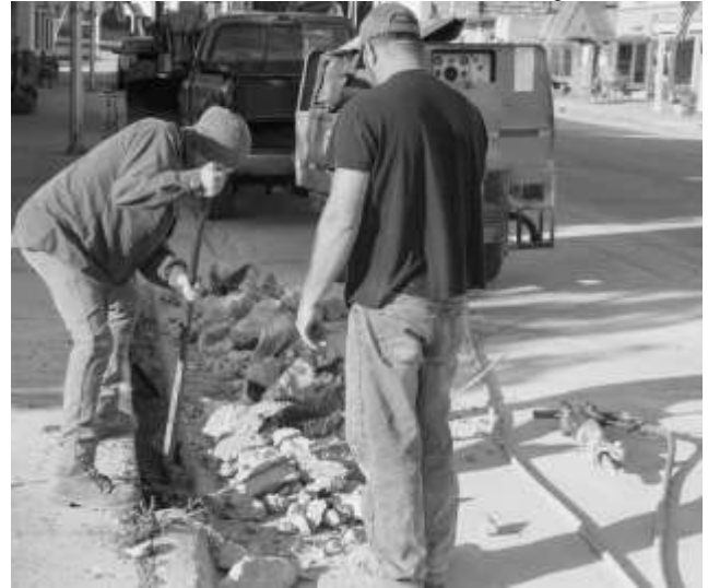
Curb and sidewalk repairs were made this summer.
